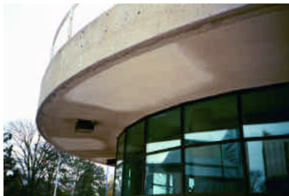
N17-P_AP5 South soffit
