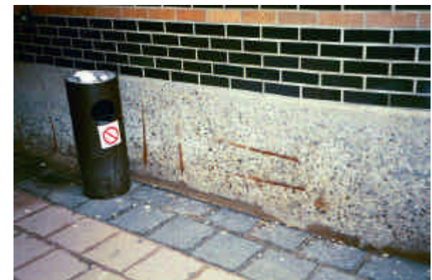
N17-P_AP6 Wall by north entrance doors
