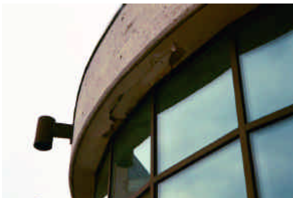
N17-P_AP4 North soffit
