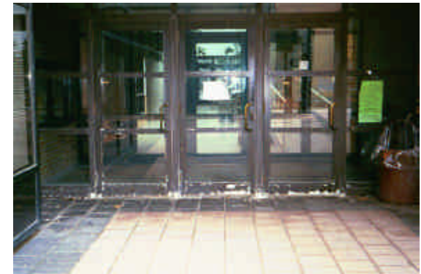
N17-P_AP3 Entrance doors
