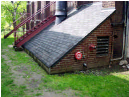
S02_AP10 Roof above mechanical room.
