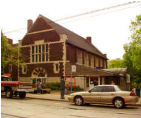
S02_AP01 North façade
